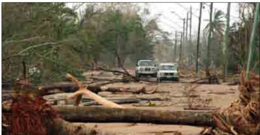
The Bruce Highway blocked after a tidal surge hit the town of Cardwell following Cyclone Yasi crossing the coast. Photographer: Lyndon Mechielsen
