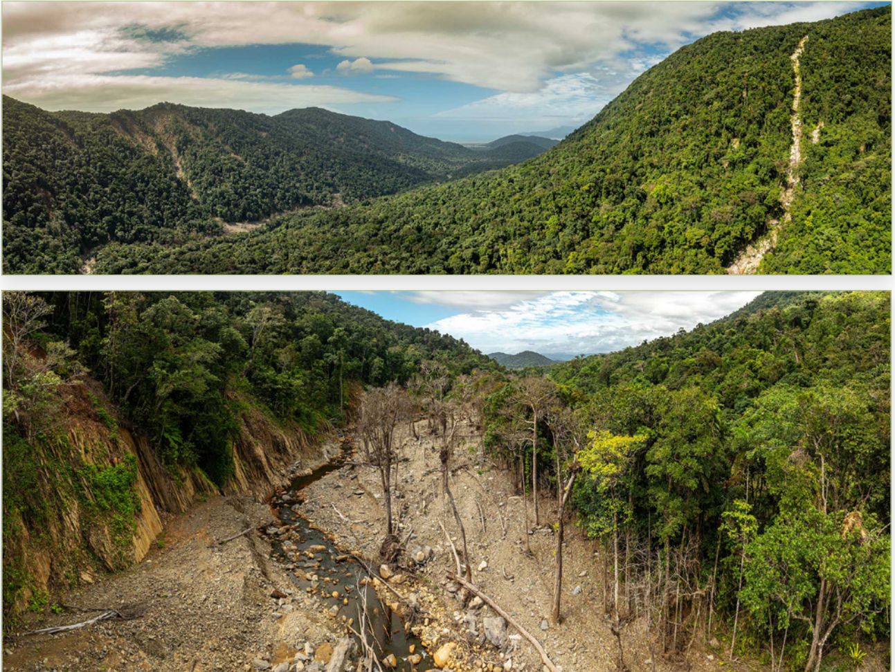
Cyclone Jasper damage. Coastal cyclone damage at Gap Creek, Eastern Kuku Yalanji Country in the aftermath of Tropical Cyclone Jasper-associated flooding in late 2023—Wet Tropics Images/Paul Curtis
