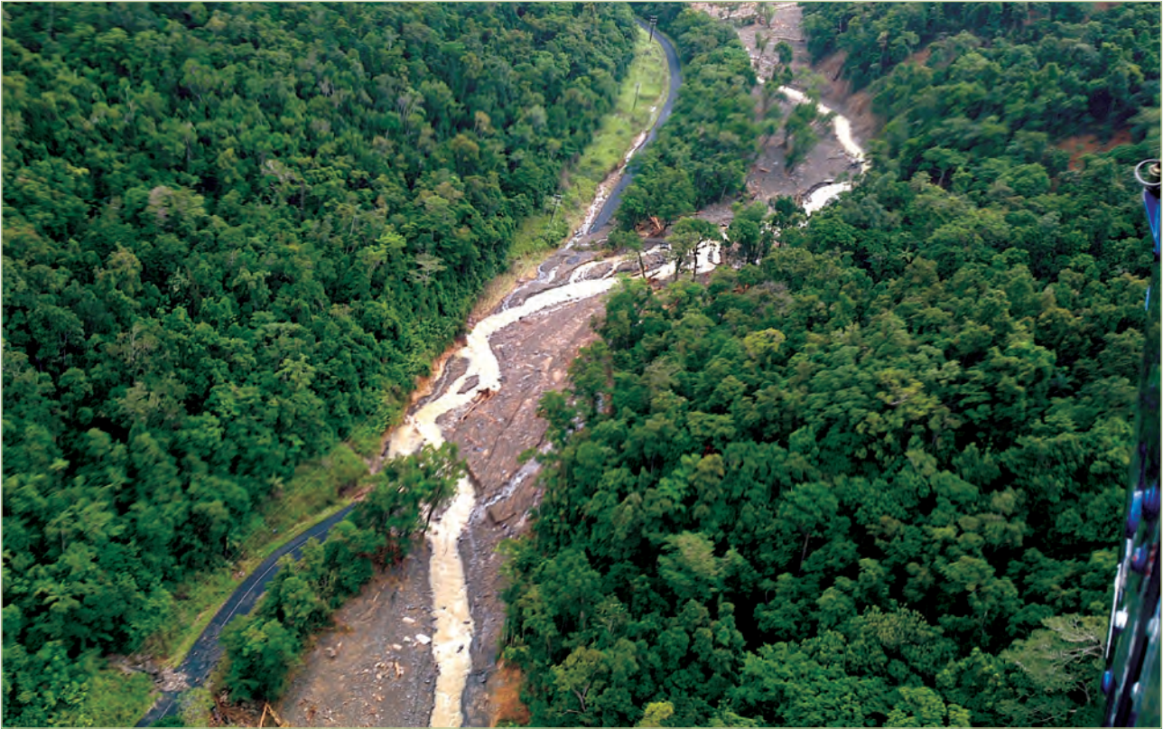
Impacts to infrastructure and access along Bloomfield Road, Eastern Kuku Yalanji Country— Cook Shire Council
