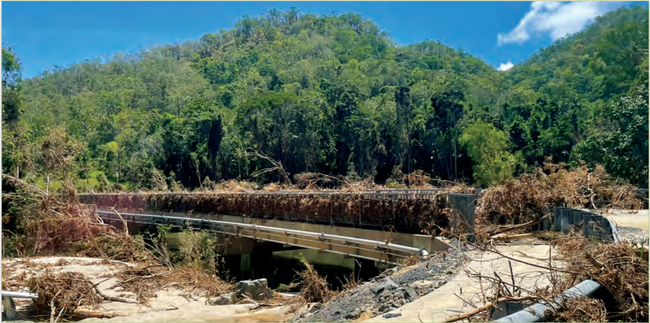
Accumulated debris across the Bloomfield Bridge at Wujal Wujal after TC Jasper. Kuku Yalanji, Kuku Nyungul and Jalunji Country—Wujal Wujal Aboriginal Shire Council
